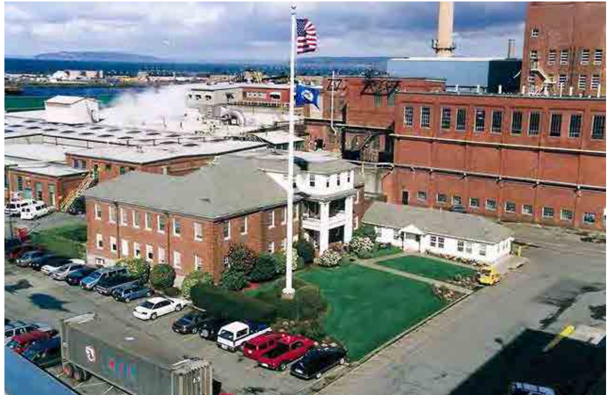
ABOVE: A circa 1990 image of Scott Paper Company and its offices, which operated on the bayfront for nearly 40 years. Kimberly-Clark purchased the 66-acre site in 1990 and began a rebuild.
