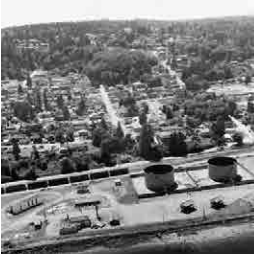
ABOVE: The northern end of the Mukilteo Tank Farm, showing two of the 10 above-ground fuel tanks.
