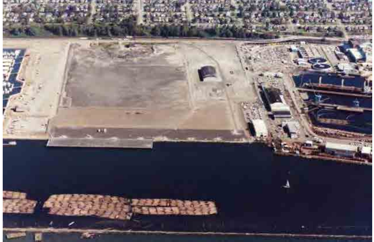
ABOVE: A 1980 aerial view of the completed first phase of the Port of Everett's newest shipping facility, Norton Terminal, located north of its larger shipping terminal site and south of the Everett Yacht Basin (now Central and South Docks). At the far north sits the vacant site that becomes Marina Village later in the decade.
