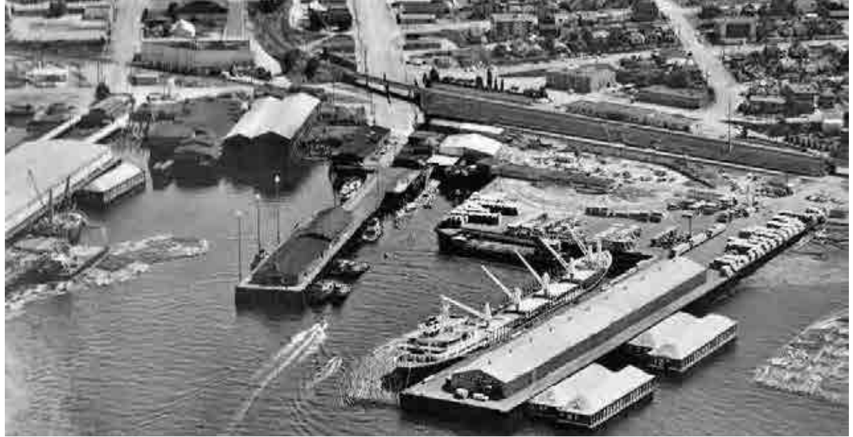
ABOVE: A circa 1968 view of the future site of the Alumina Dome beginning construction between Pier 1 (right) and Pier 2 (center); Pier 3 is shown on the far left.
